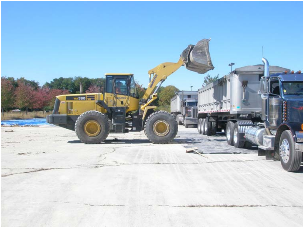
Photograph 4 – Loading Soil From Stockpiles for Disposal
