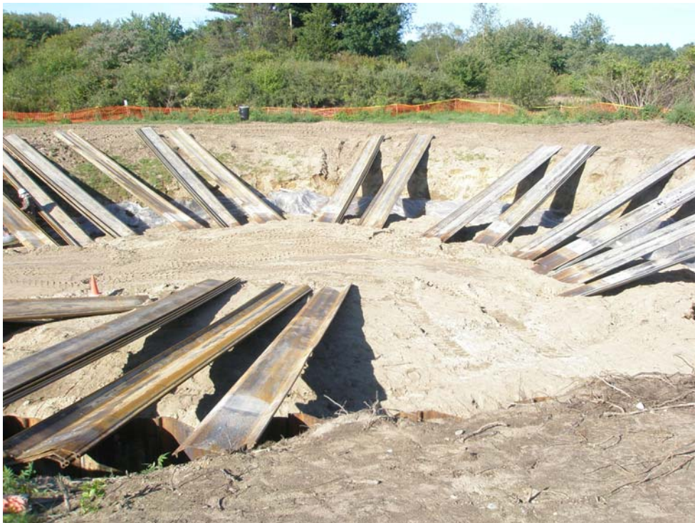
Photograph 2 – Continued Sheet Pile Removal
