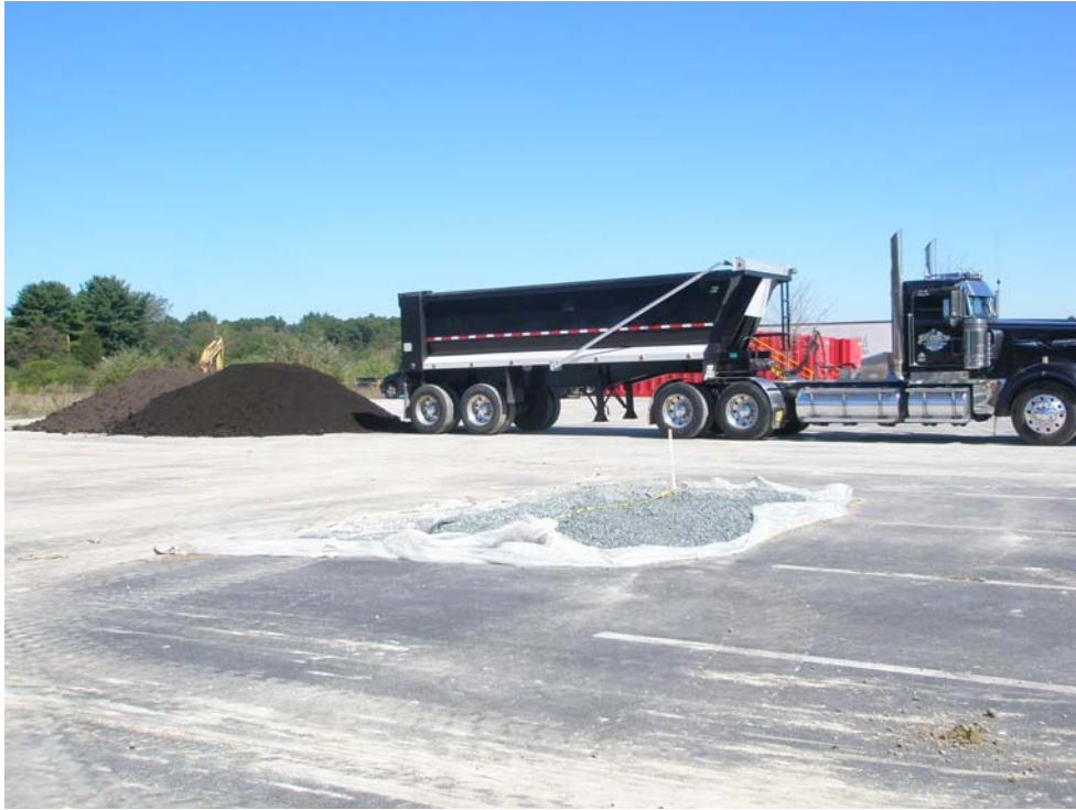
Photograph 3 – Delivery of Wetland Topsoil
