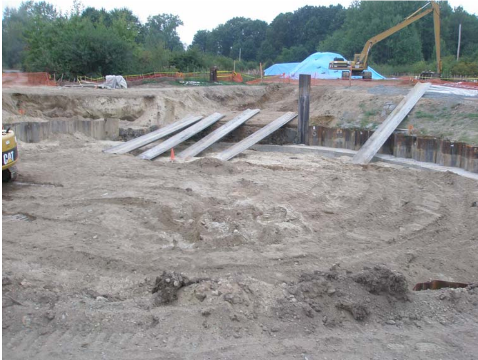
Photograph 1 – Initial Sheet Pile Removal
